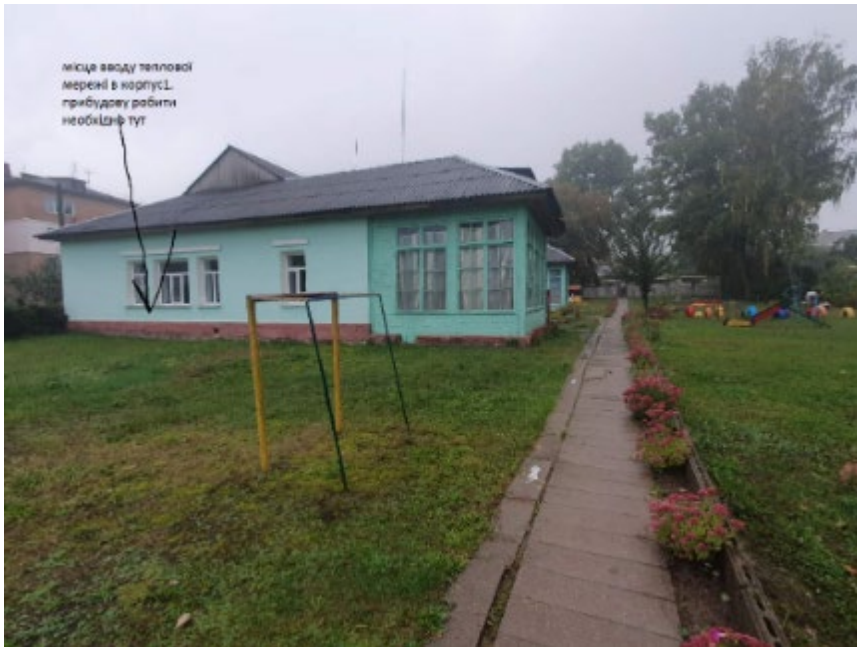
Image 1 Building 1 where an extension needed to be built.
