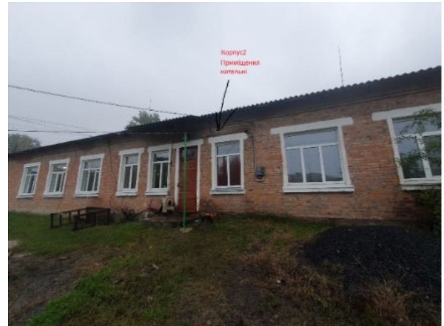
Image 2 Building 2, former boiler house facilities
