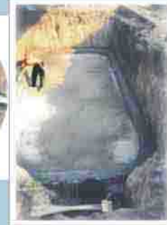
Bottom of the digester is filled with concrete taking into consideration substratum drainage during the process of processing
