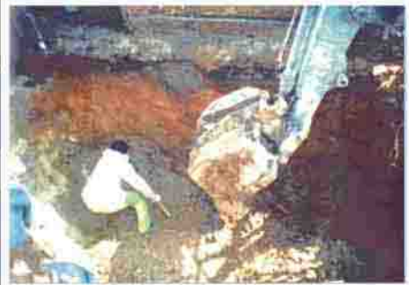
Beginning of the construction—digging of a trench
