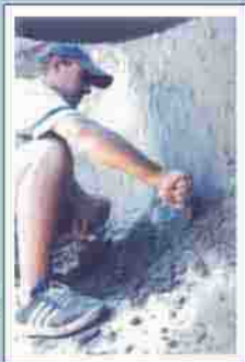
After erection the setting is thoroughly targeted
