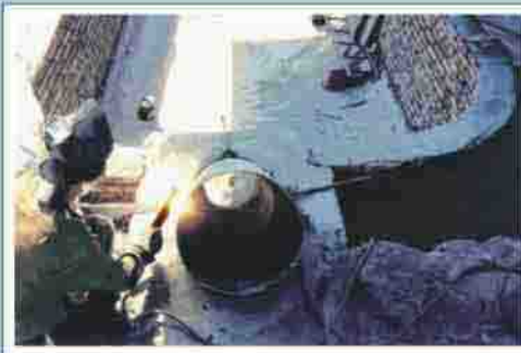
Montage of input pipe.
