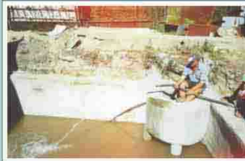
Checking of impermeability of digester's tank
