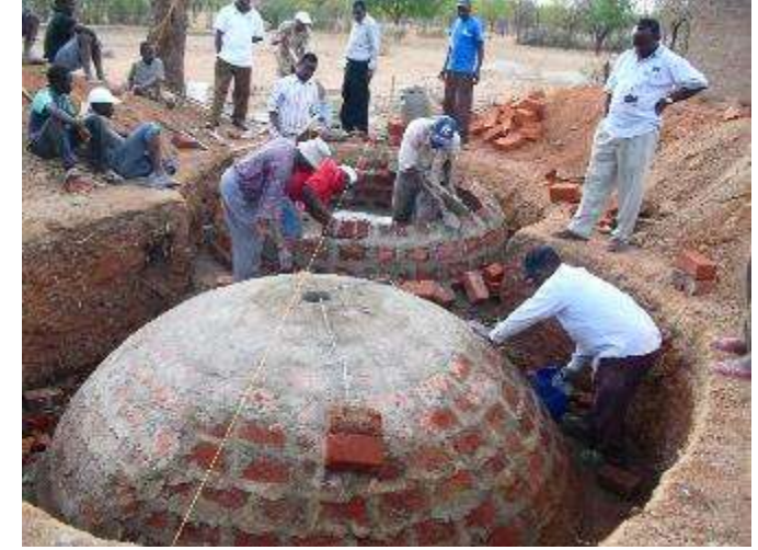
Fixed dome biogas digester
