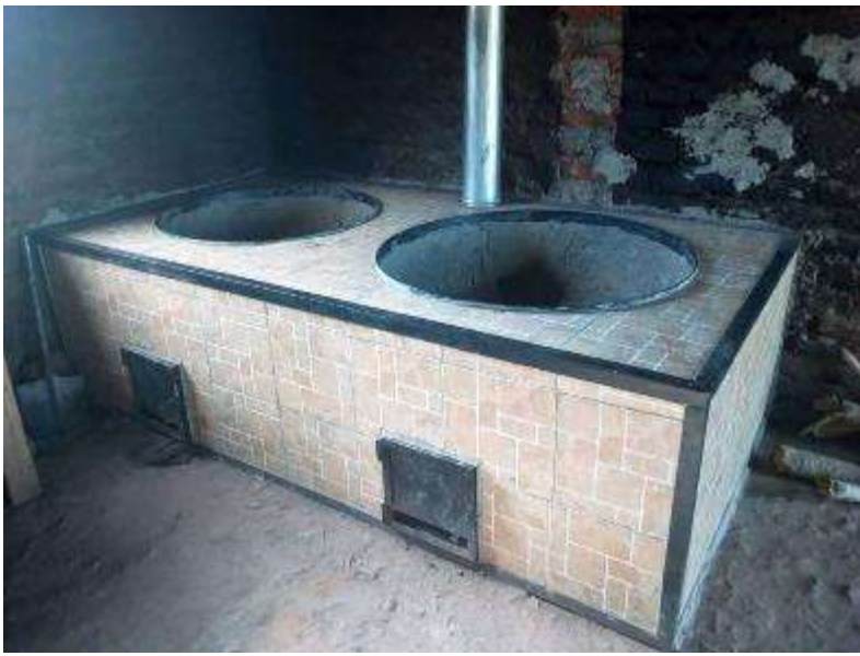
Fixed Institutional firewood stove
