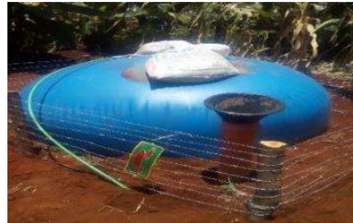
Takamoto Baloon biogas
