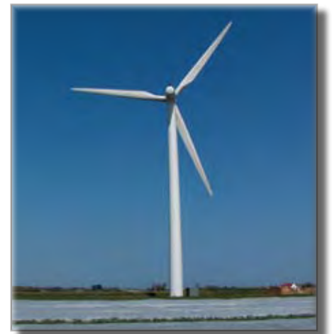
Wind mill on Samsø, Denmark
