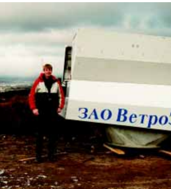
Dag A. Høystad standing beside the 200 k-W second-hand plant just before it has been erected on a hill visible from the city of Murmansk. The electricity produced by the turbine will be partly consumed by the hotel, and partly sold to the local grid.
