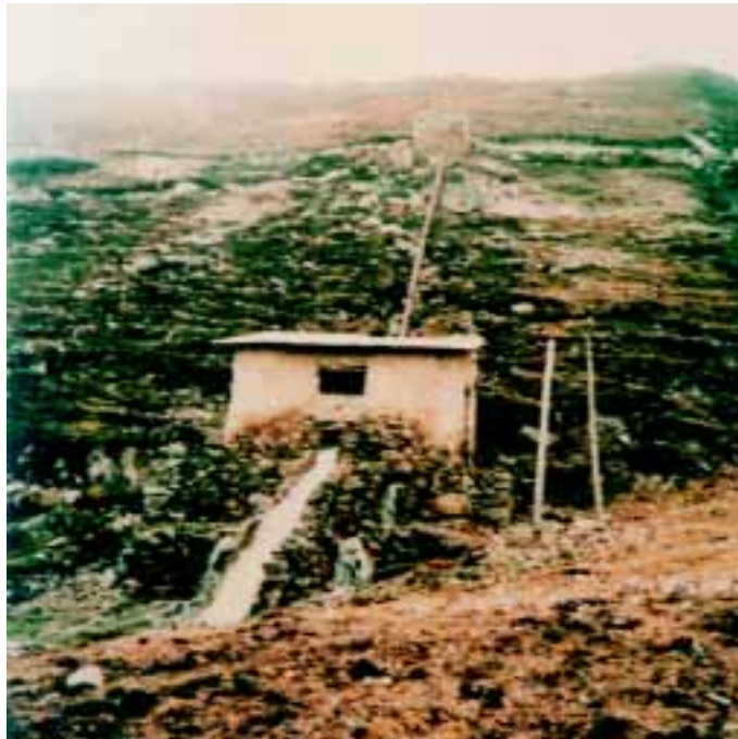
The first 6-kW prototype of the power controller developed by Steen Carlsen. The power house was built by the villagers of Quico 4,000 m high in the Andes in Peru.
