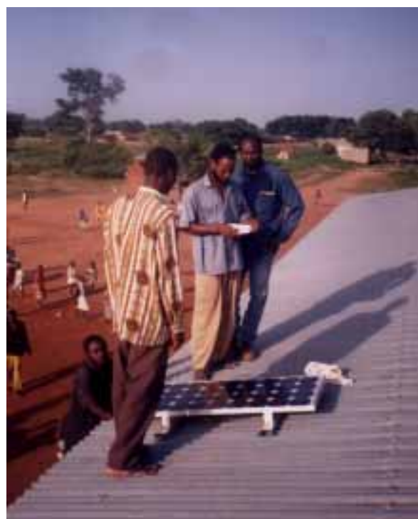
Malian Folkecenter installing a 75W solar power system for the electrification of the school in the village of Tabakoro. It now provides lighting for evening classes in adult literacy
