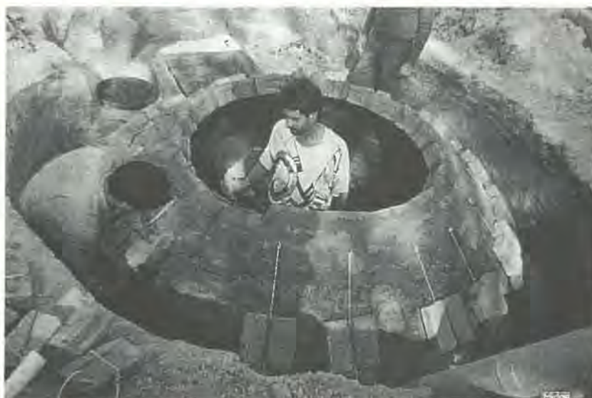
Deen Bandhu Biogas plant under construction in India.
