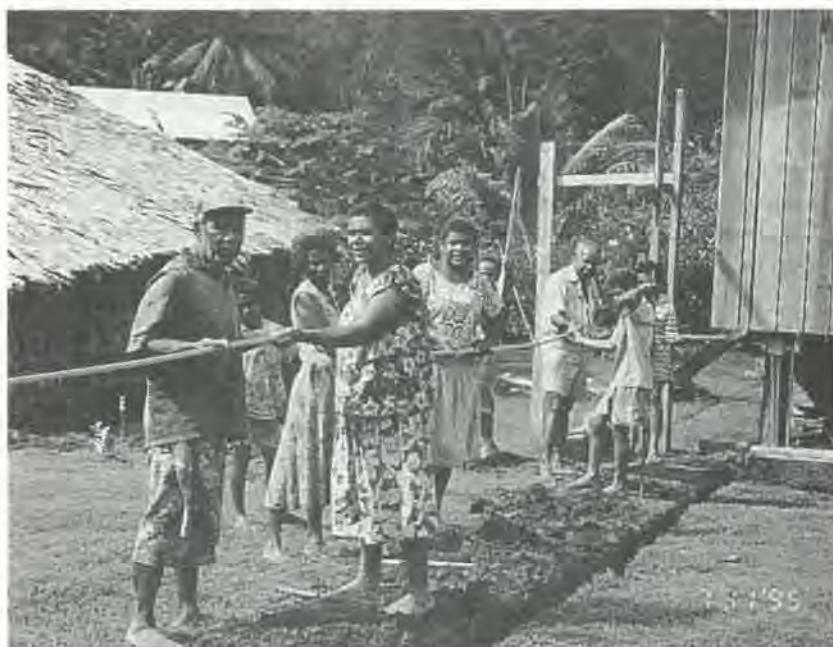
Community wiring team. Micro-hydro power is being installed. Solomon Islands.
