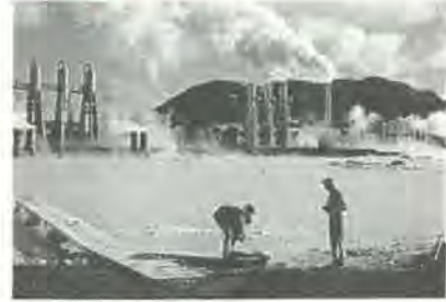
Geothermal power plant.
