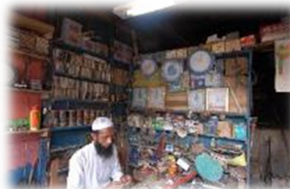
Solar System for village shop
