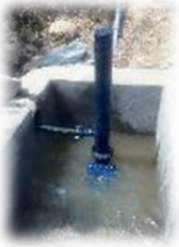
Hydraulic Ram Pump (Hydram)
