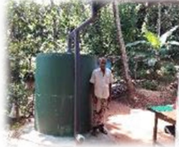
Roof rainwater harvesting.
