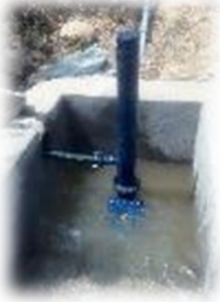
Hydraulic Ram Pump (Hydram)
