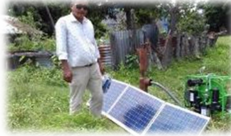
SF2 Solar Water pumps
