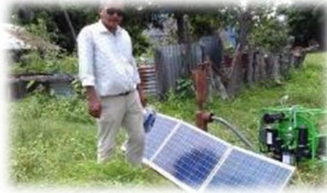
SF2 Solar Water pumps
