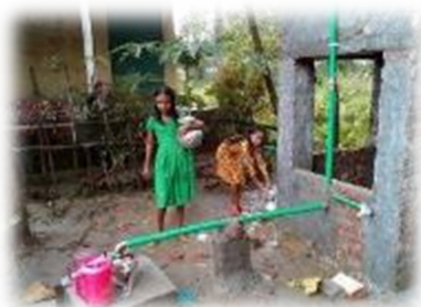
Rainwater Harvesting System
