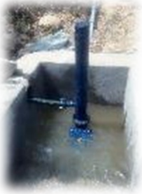
Hydraulic Ram Pump (Hydam)
