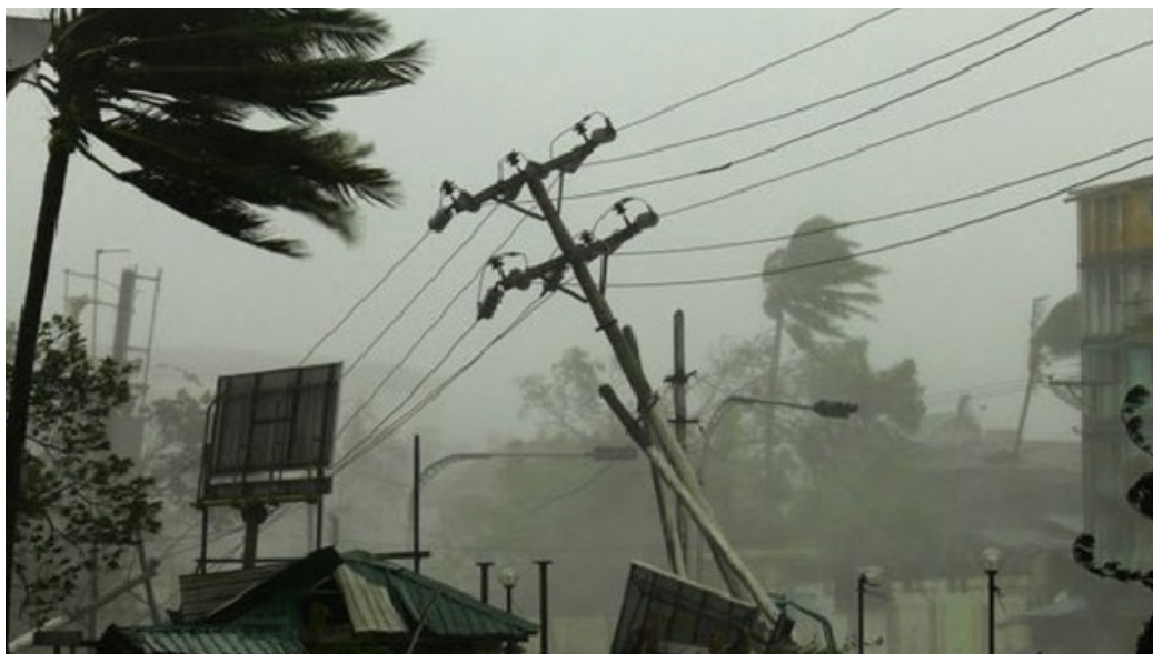
Electric poles devastated due to cyclone
