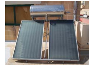
A photograph of a Solar Water Heater on top of a roof in Malta
