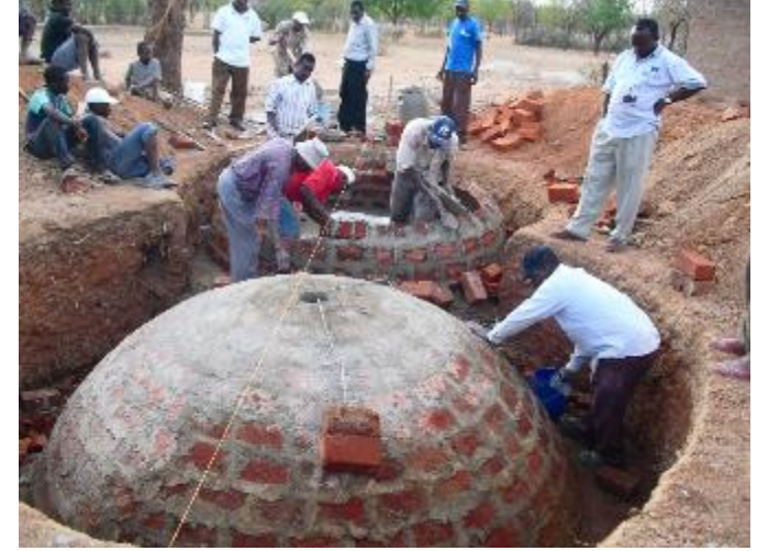
Fixed dome biogas digester
