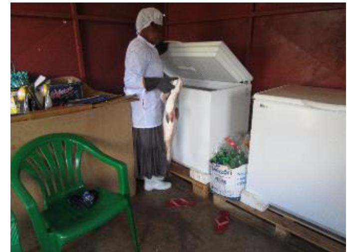
Solar Powered Refrigerator
