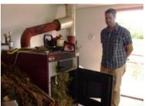
The biodiesel CHP motor is 4.5 kWh, and uses 2 liter oil/hour. It is using used vegetable oil, which is collected by the school children from their homes. The vibration is decreased by a rubber basement, and double-layer windows are decreasing the noise.
