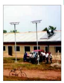
PV panels provide electricity, and solar collectors provide hot water at a health center. Photo by Youssef Arfaoui, FED.
