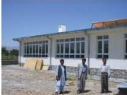
*Insulation significantly cuts the heating needs of the 1091-m<sup>2</sup> district hospital (above) in Ali-Dehe-Baba, and in the 522-m<sup>2</sup> passive solar school (below) in Lagmani, there is no need of heating. Both buildings are 1600 m above sea level.*
