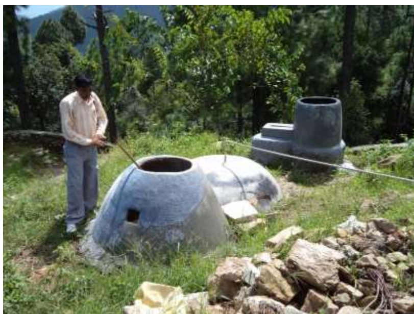
Photo: Household biogas plant (India) with inlet to the right, digester in centre, and outlet to left. Photo by INSEDA.
