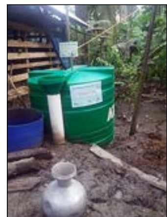
Biogas plant in Majherchar Village.
