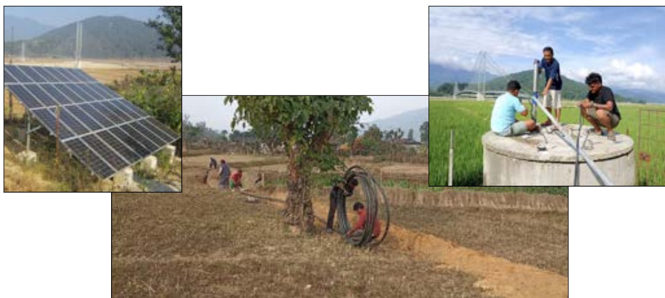
Solar powered multi-use system (MUS) for water lifting. Photos by CRT/N
