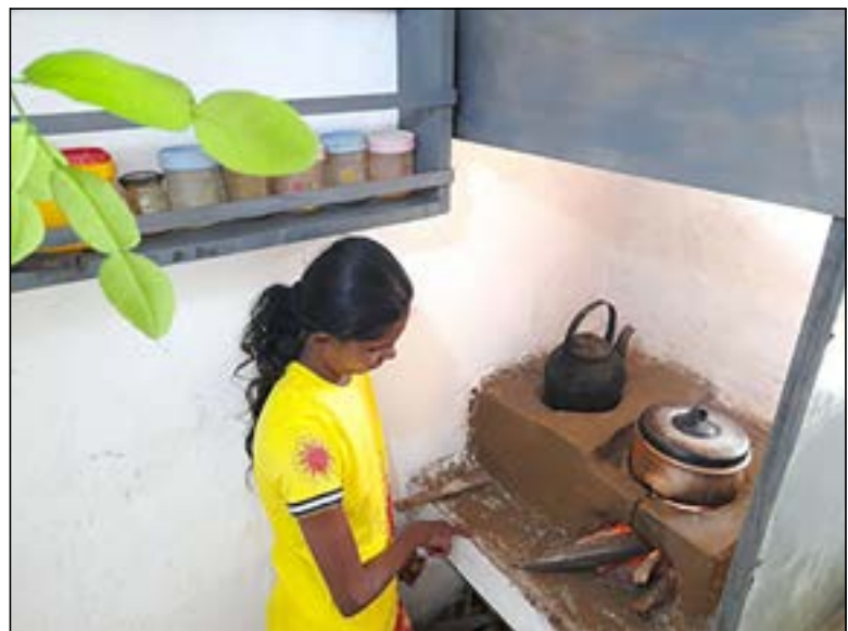
Household inbuilt Improved Cookstove (Anagi) with chimney hood installed in the village. Photo by IDEA
