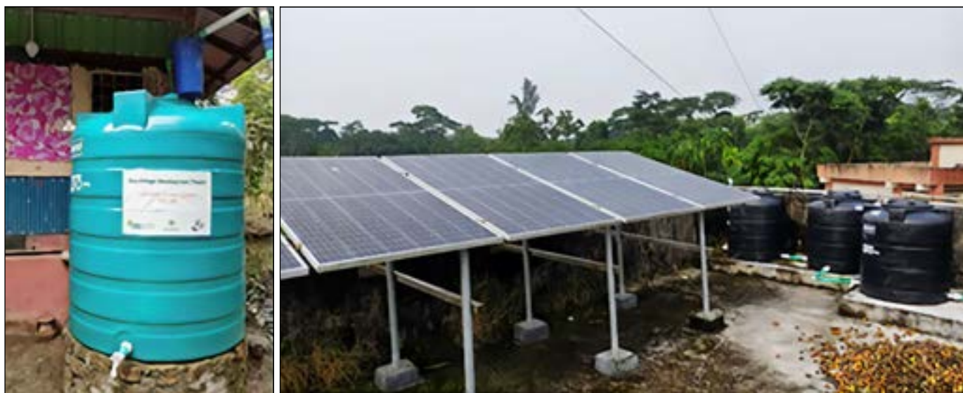
Biogas tank and solar-powered water pump installation. Photo by Grameen Shakti
