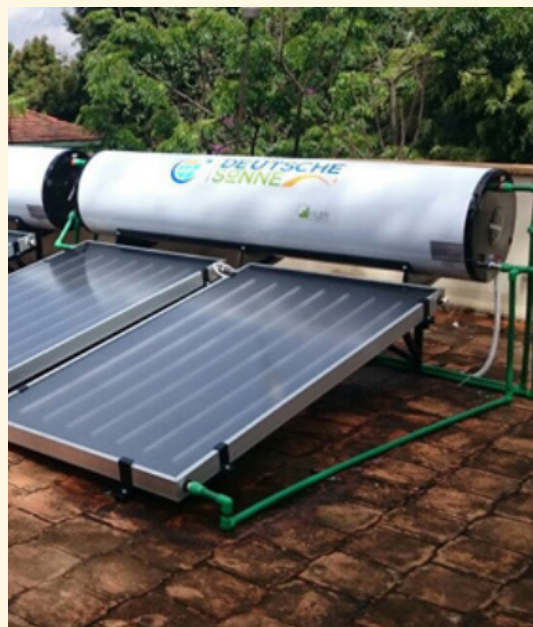
Direct Solar Water heater (Lean Energy Solutions, Kenya)
